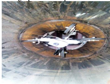
Photograph 6.3 PIR locating defects
